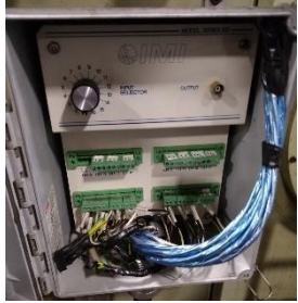
Top : IoT Hub Bottom Left: Accelerometer junction box Bottom Middle: Interconnect Bottom Right: IEPE adapter
