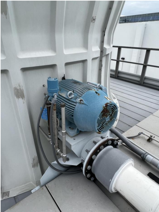
Image 2: Cooling Tower Motor
